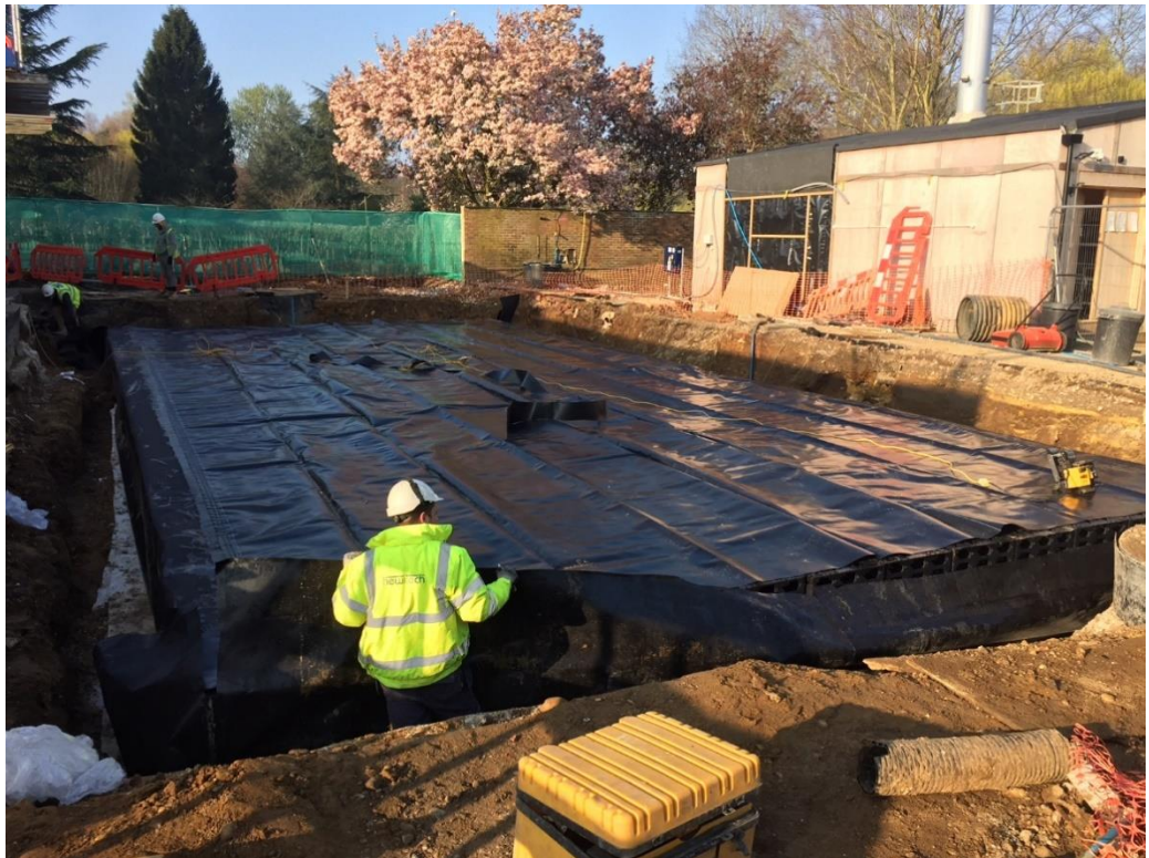
Photo 2: Part of SUDs system being installed
