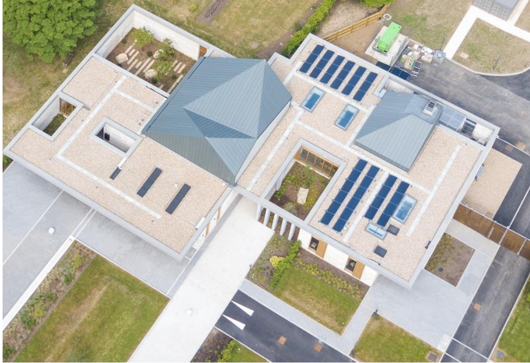
Photo 3: PV array on roof of new building (Credit Dan Hannington)
