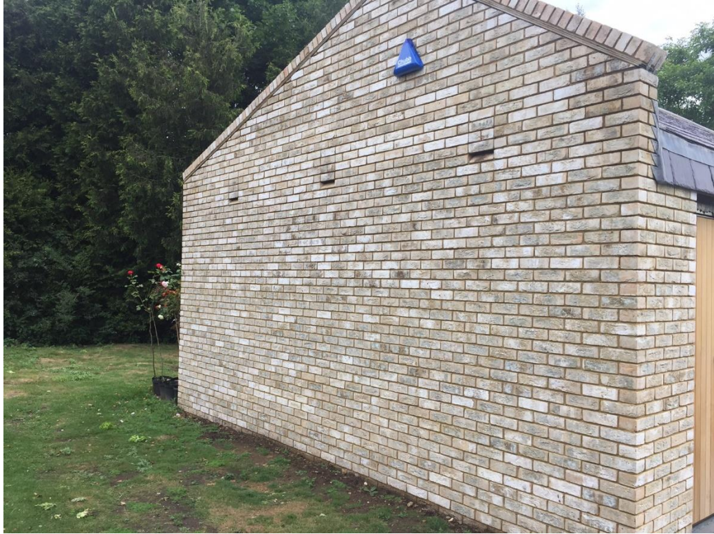
Photo 1: Bat bricks in groundsman store to provide replacement habitat
